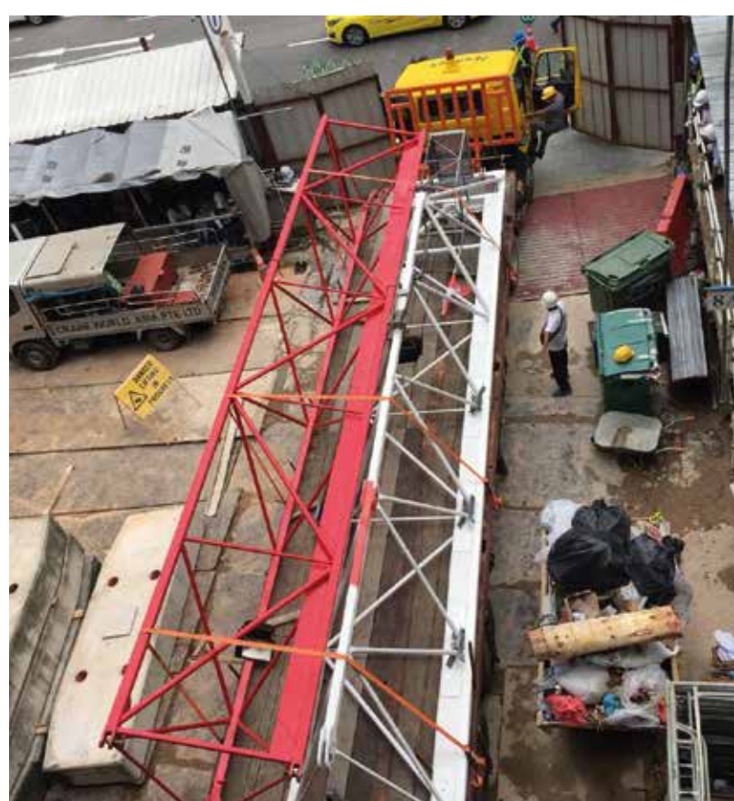
Tower crane dismantling
