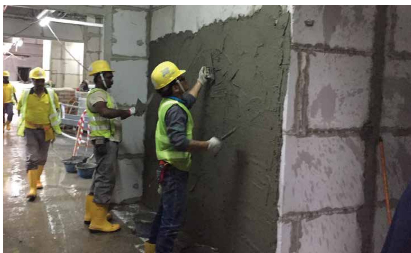
On-going plastering works
